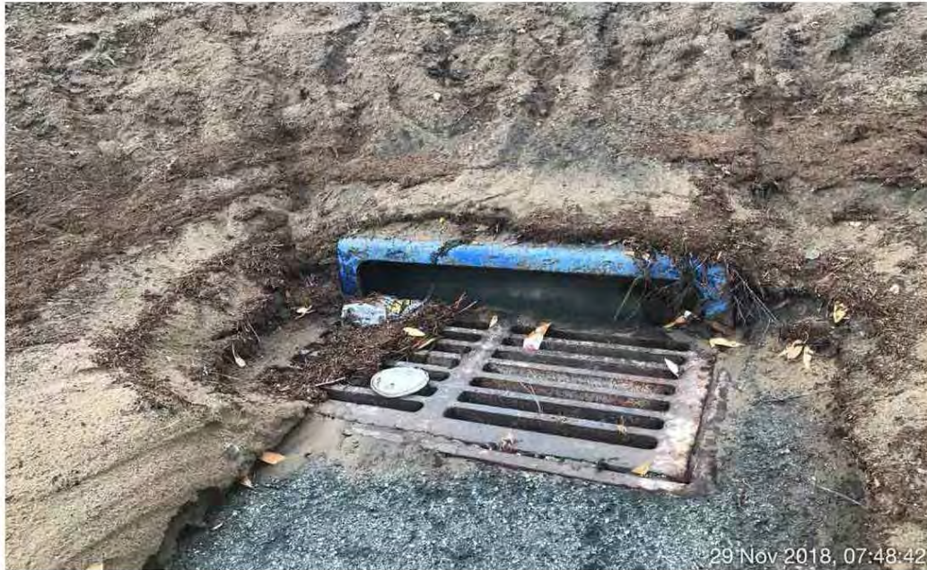
Photo 6. High water mark at pond outlet structure, 11/29/18
