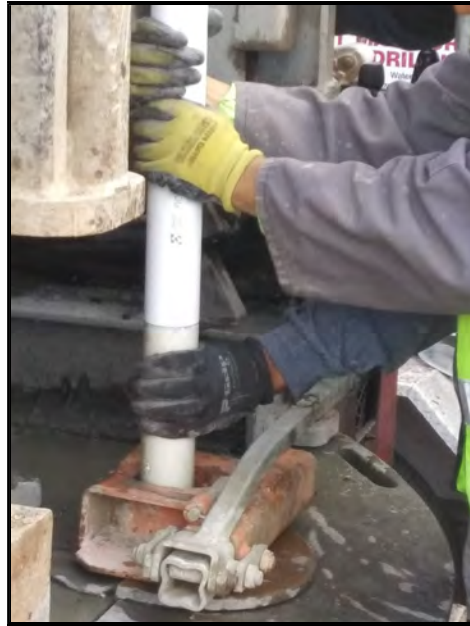
Installing the 2" Schedule 80 PVC Casing. The joints are flush threaded.
