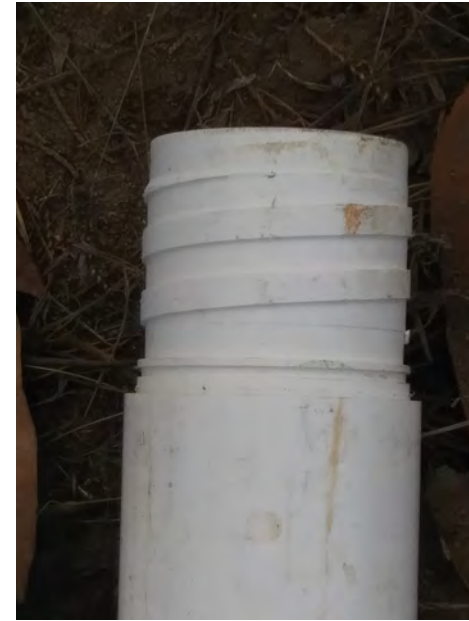
Installing the 2" Schedule 80 PVC Casing. The joints are flush threaded.
