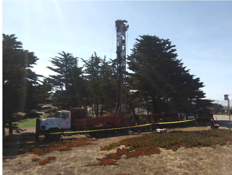
Photos of the drill rig
