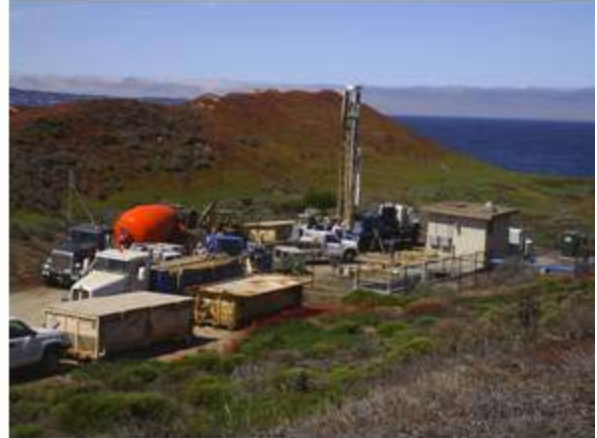
Drilling Operations at SBWM #4
