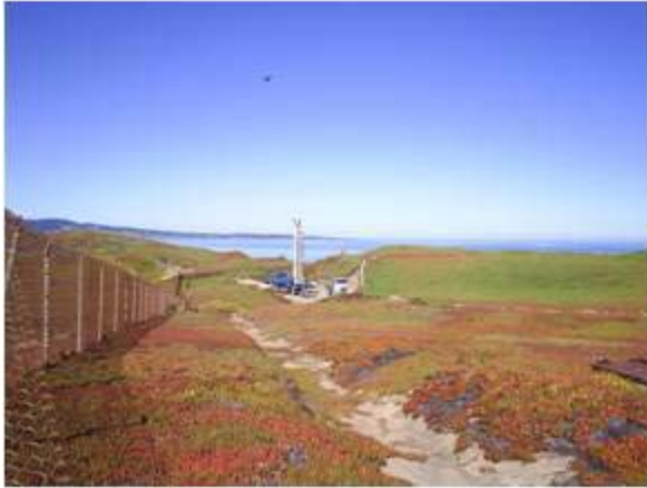
Drilling Operations at SBWM #3
