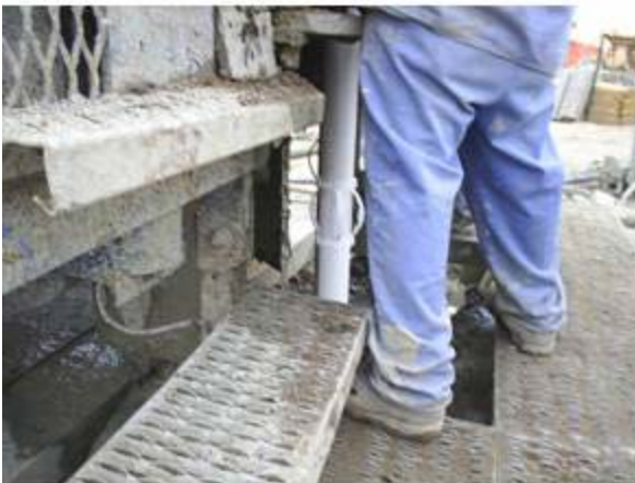
Casing Installation w/ Centralizer
